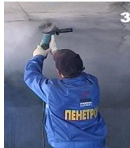
Make U-shaped indents along the whole length of the cracks, seams, joints, couplings and junctions and around all service line entries. Clean the indents with a wire brush. Remove the loose concrete layer (if any). Using a jackhammer, rout out the cavities of the pressure leaks to a width of 25 mm or more and to a depth of 50 mm or more, making them wider towards the interior (if possible, in the shape of a dovetail). Remove the loose, peeled off concrete from the inside of the leak.
